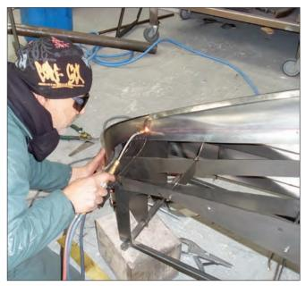
Butt-welding two panels together on a fender by hand using a gas or oxygen-acetylene torch and minimal heat. (*David Cooper*)
